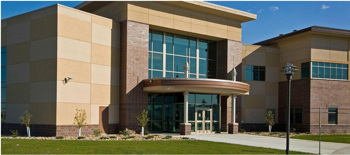
Figure F.20.1: Cass County Electric Building
