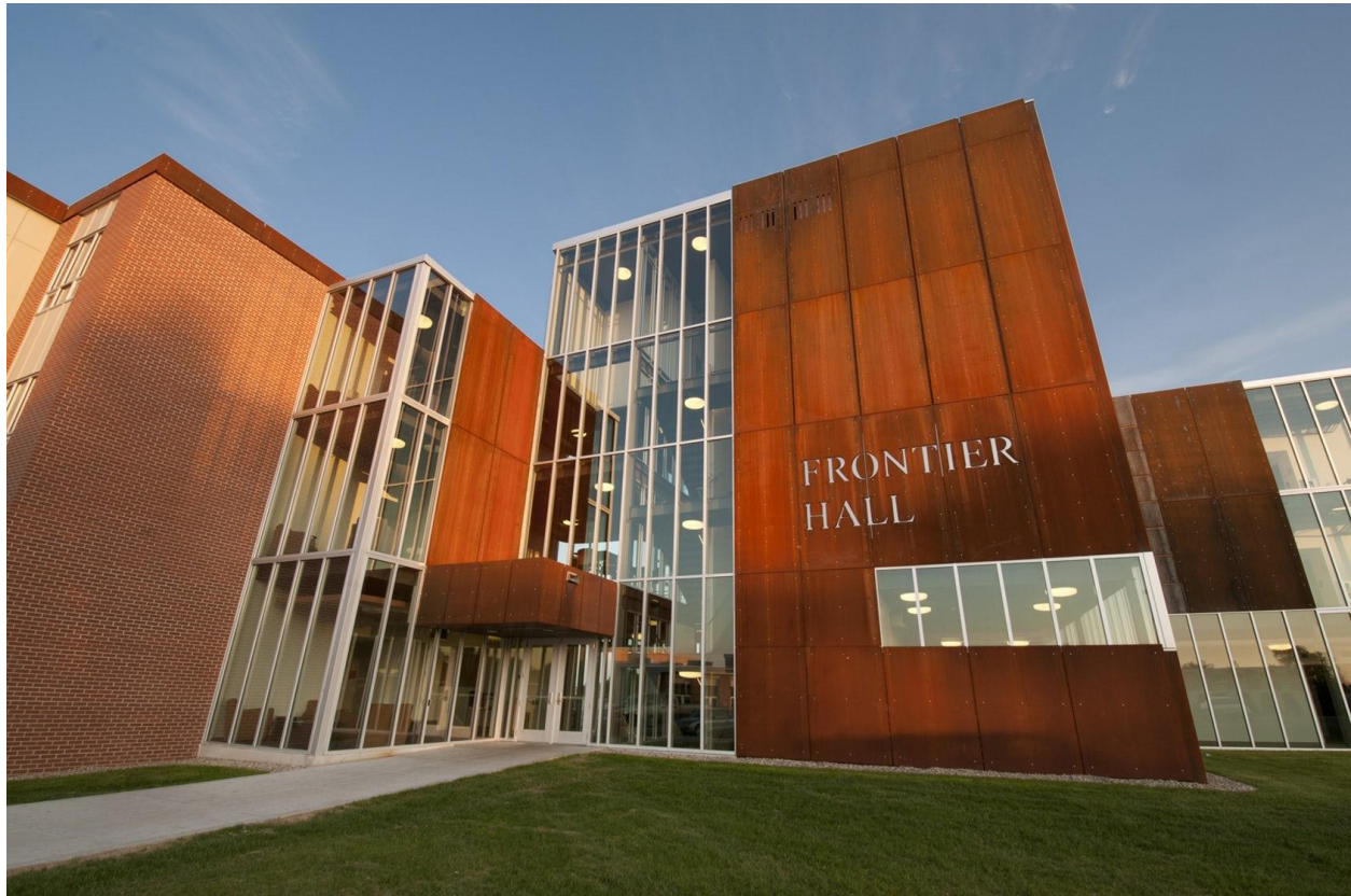
Figure F.9.1: WSC Frontier Residence Hall
