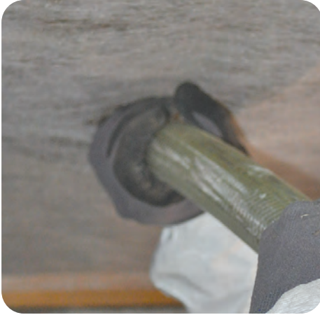
13. Loose fill netting to required density
