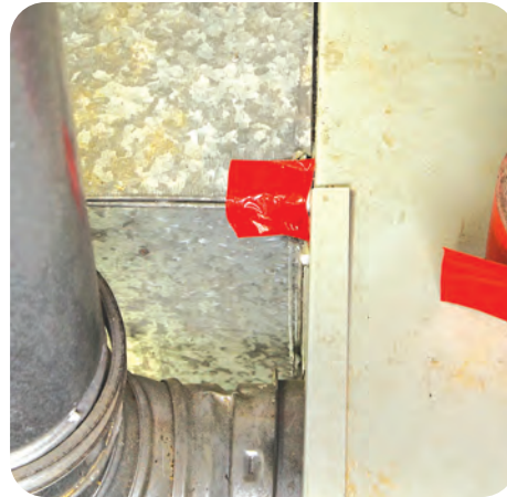
B-2. Apply temporary tape as a backer to hold mastic
