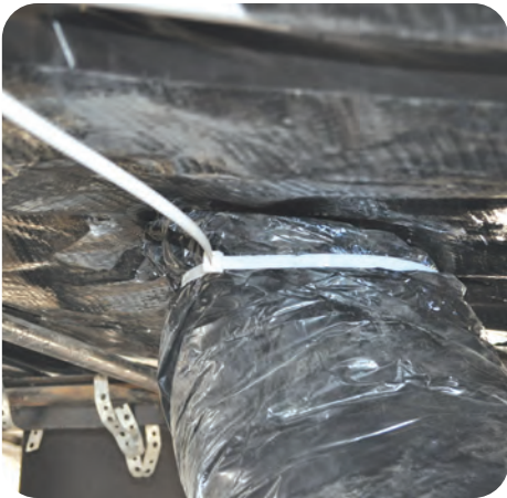
3. Secure vapor retarder layer at boots
