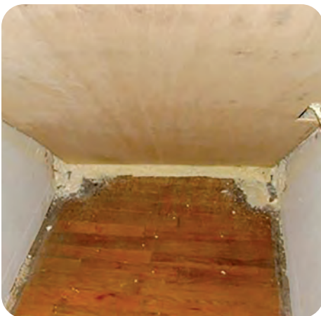
10. Seal off insulation from conditioned space in home
