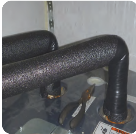
Insulation should be continuous with no gaps
