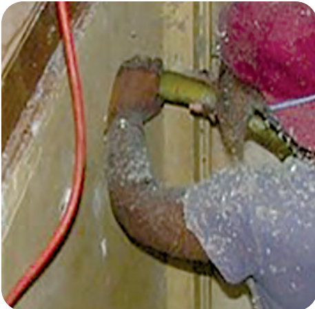
7. Dense pack stairway walls
