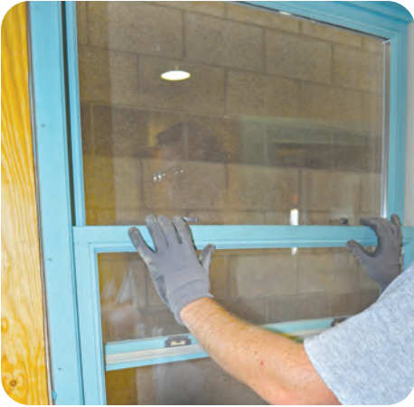
7. Ensure window is operational
