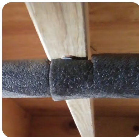
When path is partially obstructed or curved, shape insulation to the location to eliminate gaps
