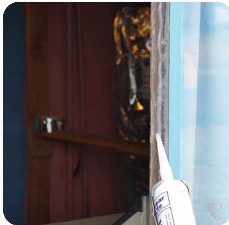
4. Run interior bead of caulk
