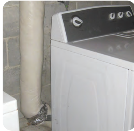
6. Duct in uninsulated space is insulated
