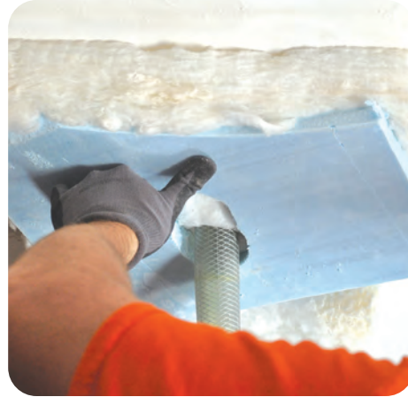
6. Blow insulation to completely fill cavities to prescribed density
