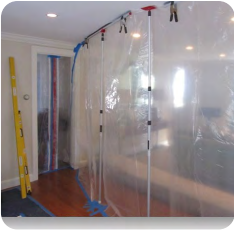
1. Protect work area from debris and dust
