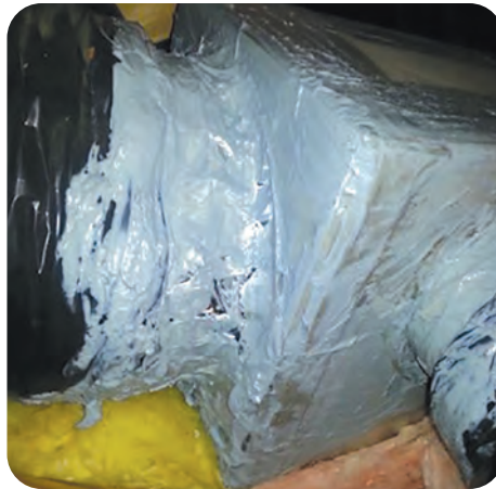
4. Seal new joints
