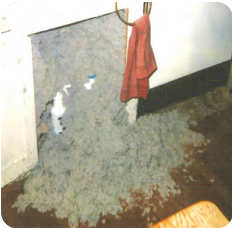
3. Ensure wall integrity is complete (no holes)
