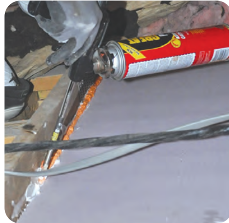
B-2. Seal around infill materials
